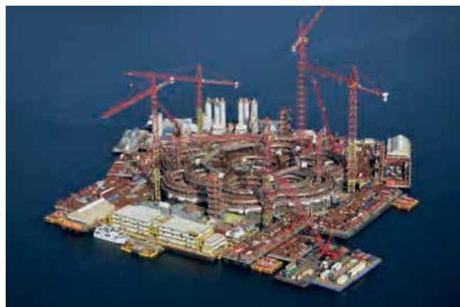
Photo: Construction of the Hebron gravity-based platform structure continued during 2014.
