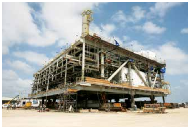
Photo: The topside modules for the Jack/St. Malo development in the fabrication yard near Ingleside, Texas.
