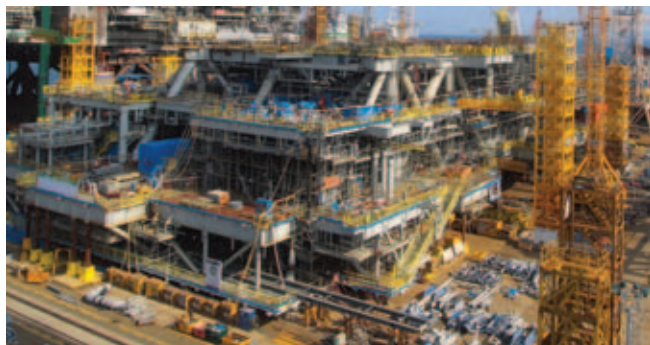
Photo: Construction of the Wheatstone platform topsides in Okpo, South Korea.
